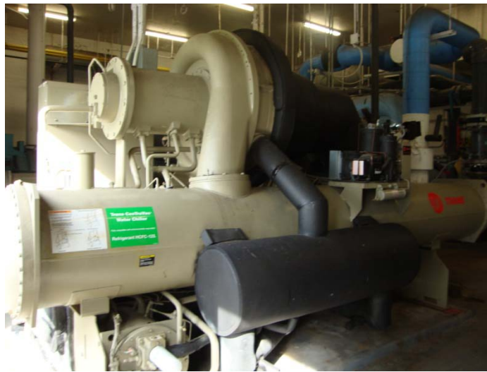
Figure 4.2.2 Water-Cooled Chiller
