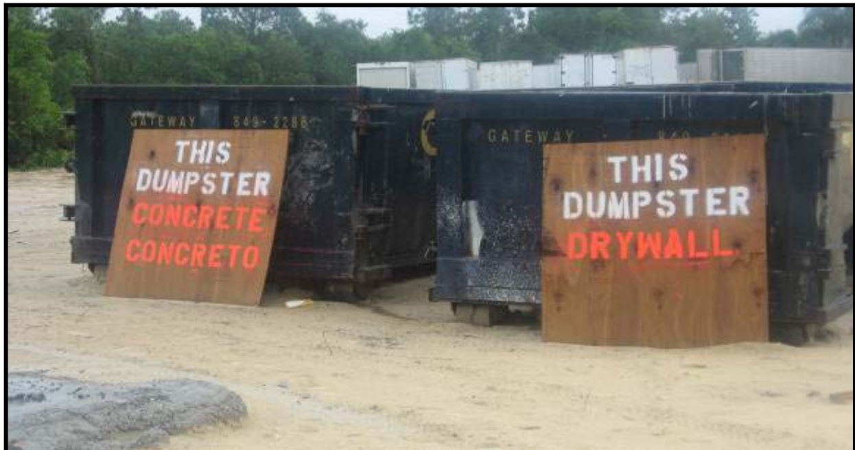
Figure 6.5 Separate dumpsters were used to facilitate the recycling of materials used on the project.
