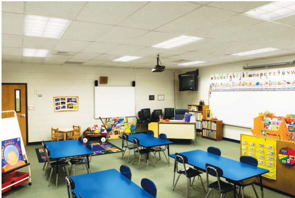
Figure 5.2 Volumetric Lighting Retrofit
