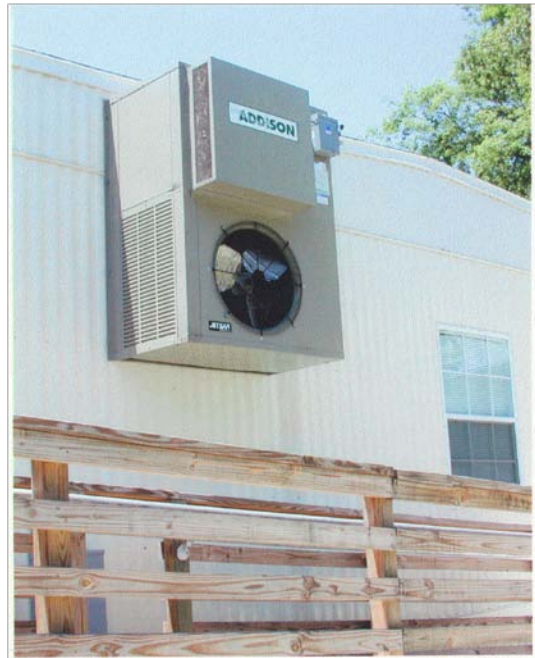
Figure 4.1.1 Wall-Mounted Unit
