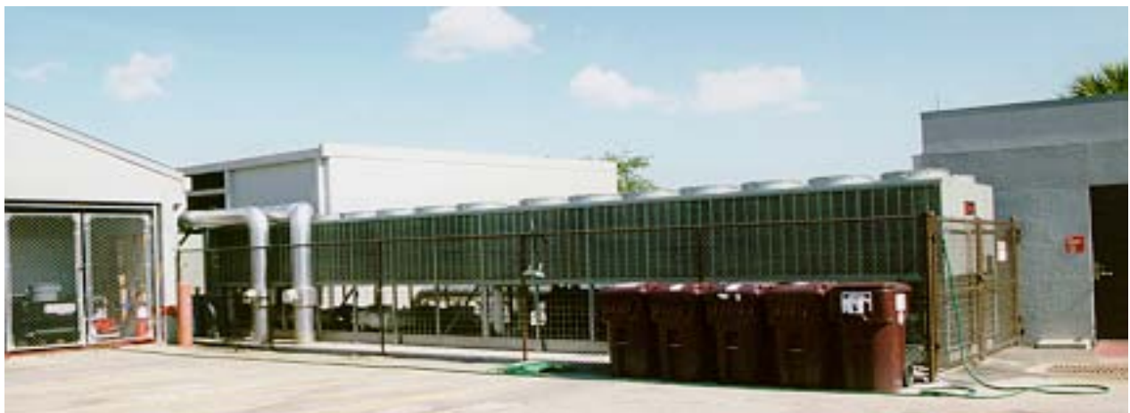
Figure 4.2.1 Air-Cooled Chiller
