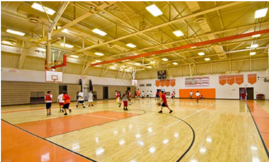
Figure 5.8 Highbay Lighting in a Gymnasium
